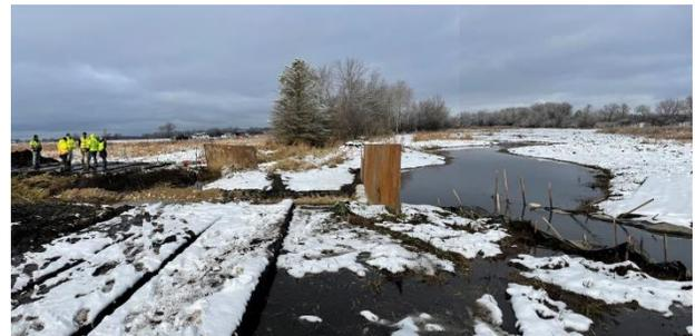
*Before “tie in” of new channel with original channel: road plates divert water away from sensitive areas through a diversion channel.*
