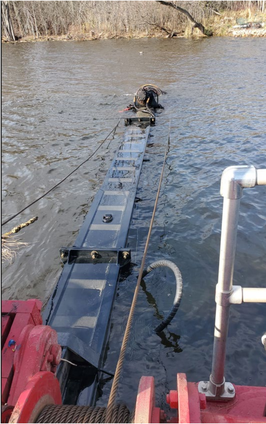
The dredge head has a 30'+ reach
